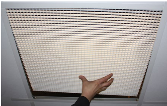
Figure 1. Installation de la grille.
