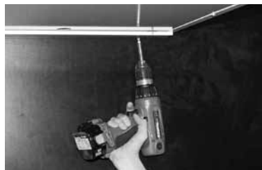
Attach the ILTO W80 to the mounting bracket by its casing.
